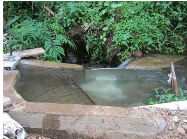
Figure 5. Dams built in the river
