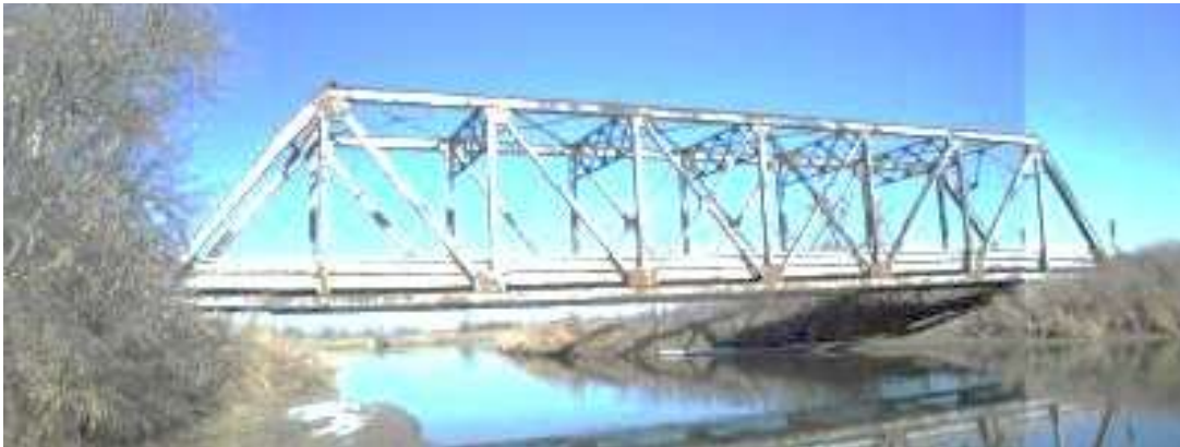
Gambar 3. Struktur jembatan sistem rangka batang ( truss ). Sumber: https://bridgehunter.com/ut/cache/5034C .
