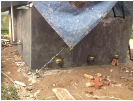
Gambar 14. Sparing pipa
